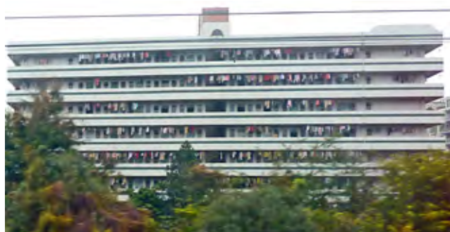
Figure 20 Many of the factories in Dongguan and Shenzhen have large dormitory buildings within their compounds where migrant workers live in crowded accommodation.
